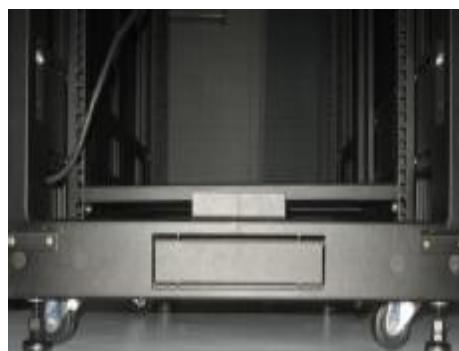
Bottom Cable Entry Access
